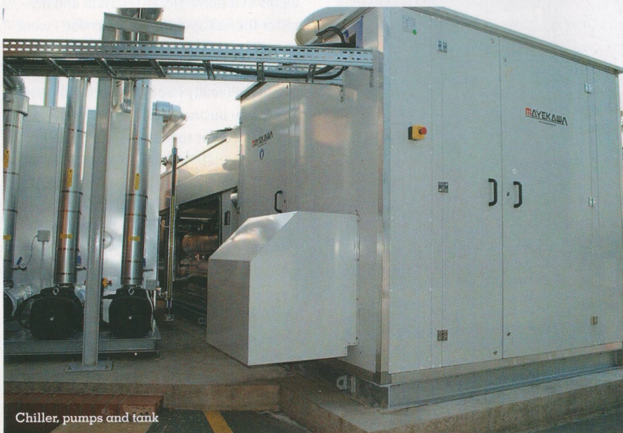
Glycol pumps and tank on site
