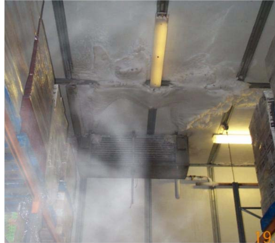
Figure 8 Frost and snow bound ceiling
