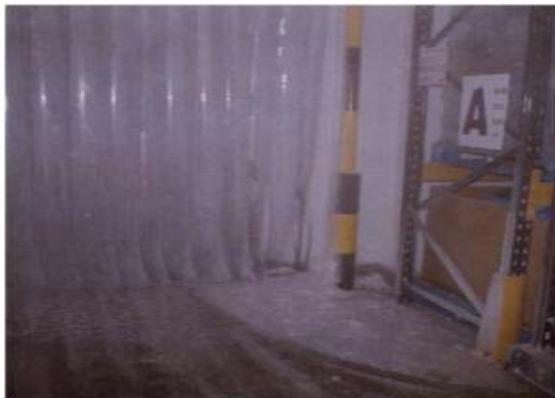
Figure 1. Snow and ice covered floor.
