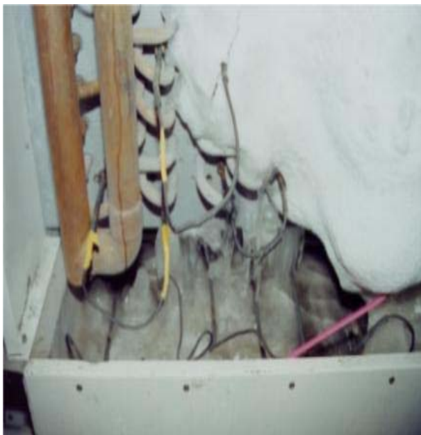
Figure 3 Iced up drip
